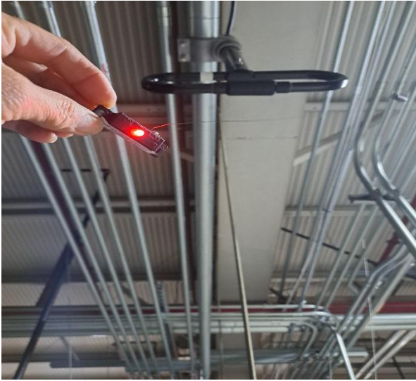
Fig.18 Testing DAS antenna system
